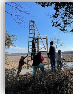
Install of box in new upland location
